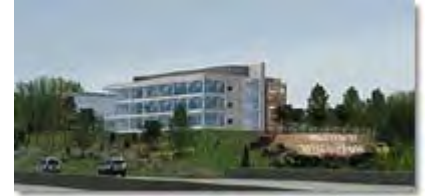
American Lung Association of Minnesota Mendota Heights, Minnesota Architects: Perkins & Will, The Weidt Group, Dunham Associates
