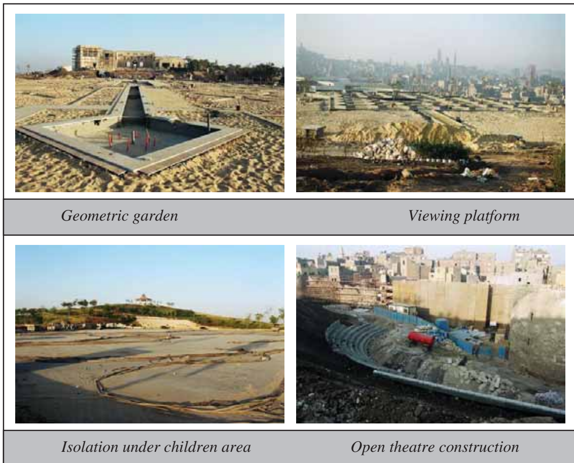
Figure 9-20: Construction stage in Al-Azhar park 30
