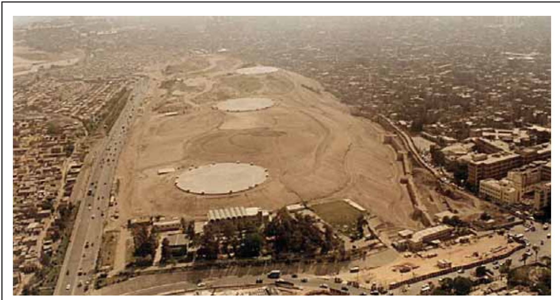
Figure 9-2: Grading in Al-Azhar Park Site to replace the existence soil 8
