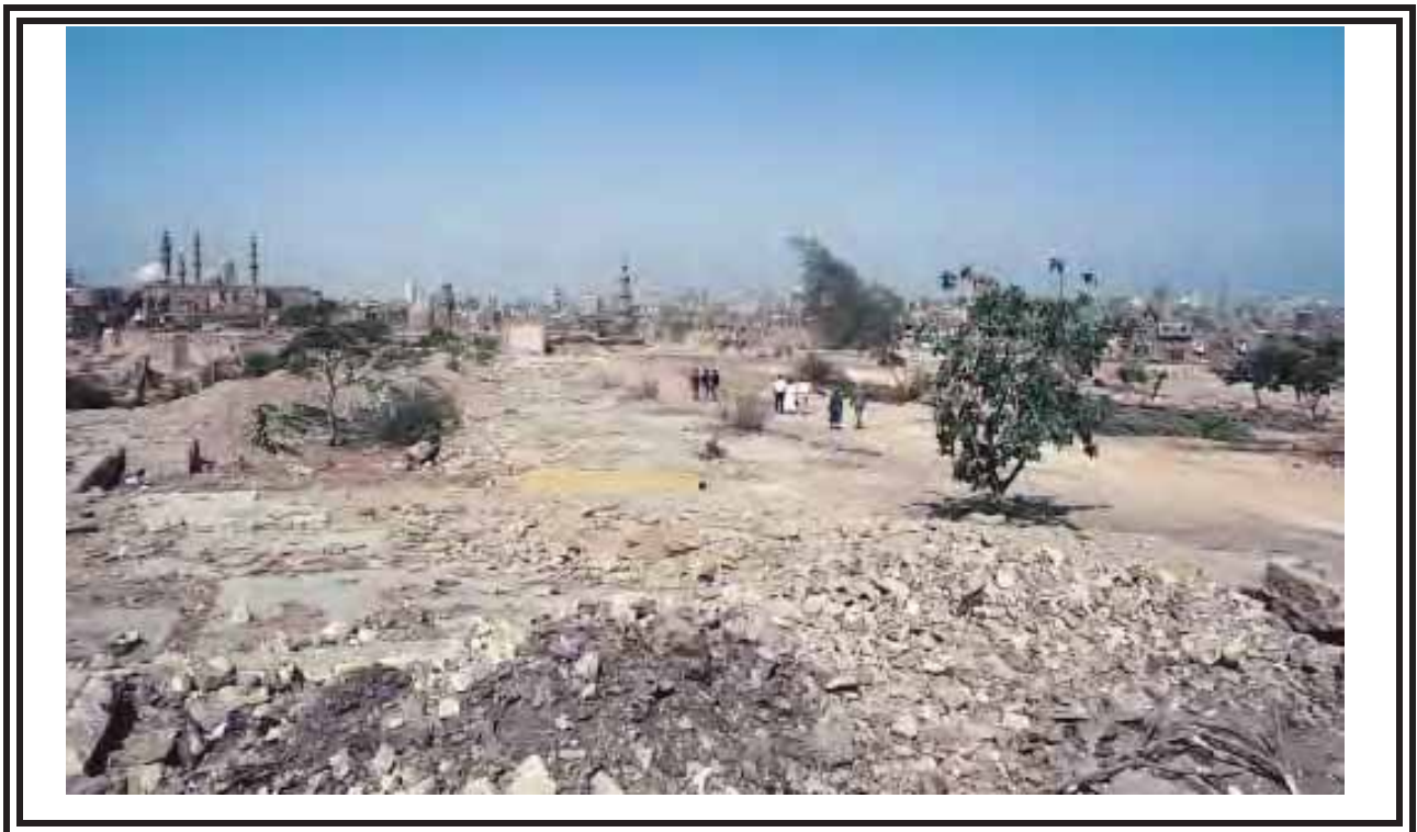
Figure 6-10 The Park site in 1992, before work commenced looking to the south. In the distance to the left is the Citadel of Salah al-Din and in the center, the minarets of the Sultan Hassan Mosque complex.
