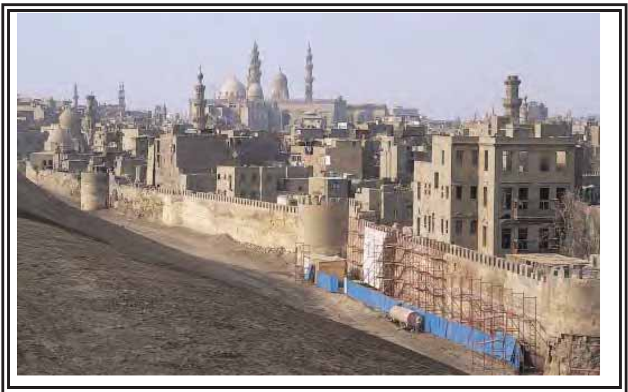
Figure 6-21 The pilot restoration project (between towers 5 and 7) under implementation.
