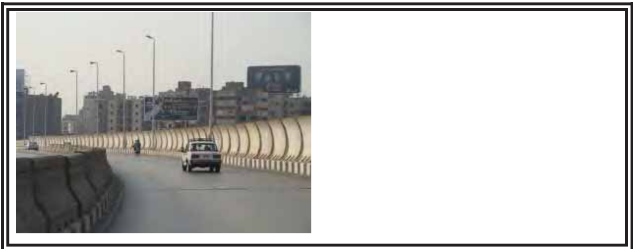
Figure 2-9 sound barriers on 6 October bridge
