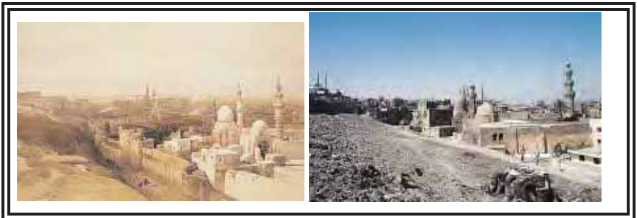
Figure 6-16 The southern section of the Ayyubid city wall and the adjacent Mosque of Aq Sunqur "Blue Mosque" and Khayrbek. first: Conditions in the 19th century (David Roberts) second: Conditions in 1992 show the wall buried beneath heaps of rubble and debris.
