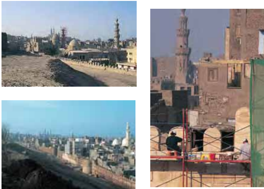
Figure 6-18 restoration for the wall
