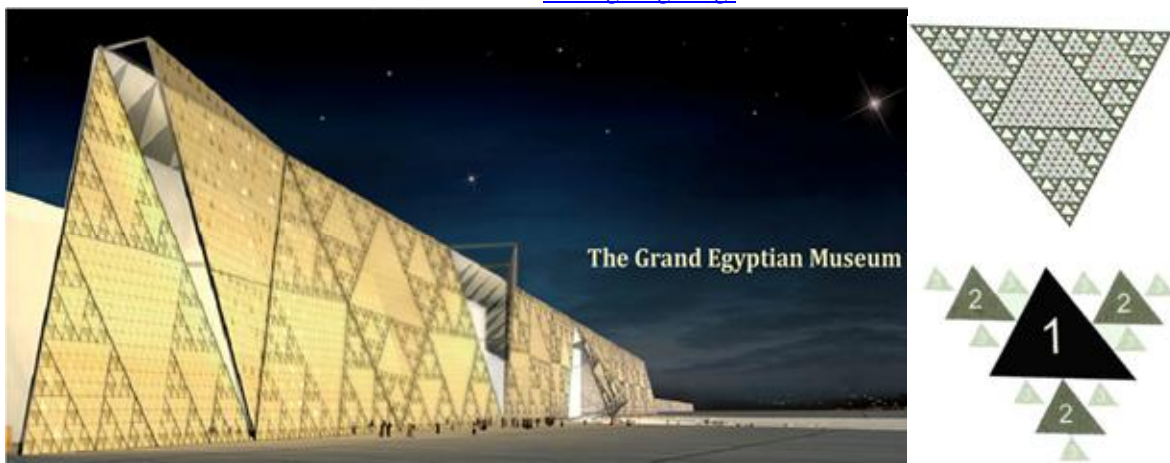
Figure 4.9 a. GEM main elevation. b. fractal arrangement on the elevation. Source: www.gem.gov.eg/
