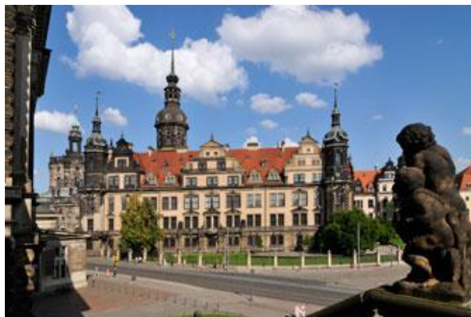
Figure1.2 Dresden palace – Germany
