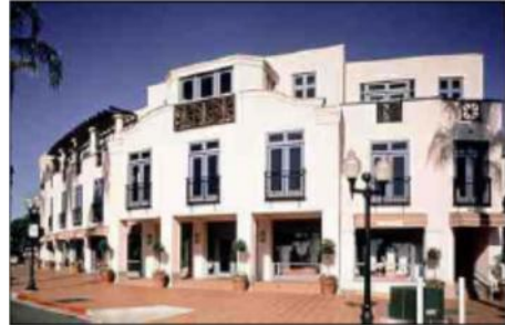
Figure 1-20: Retail, offices and upstairs residences occupy a mixed use structure. (Ewing and Hodder)
