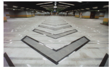
Figure 1-14: Granite Flooring in Attaba Station, Downtown, Greater Cairo.†
