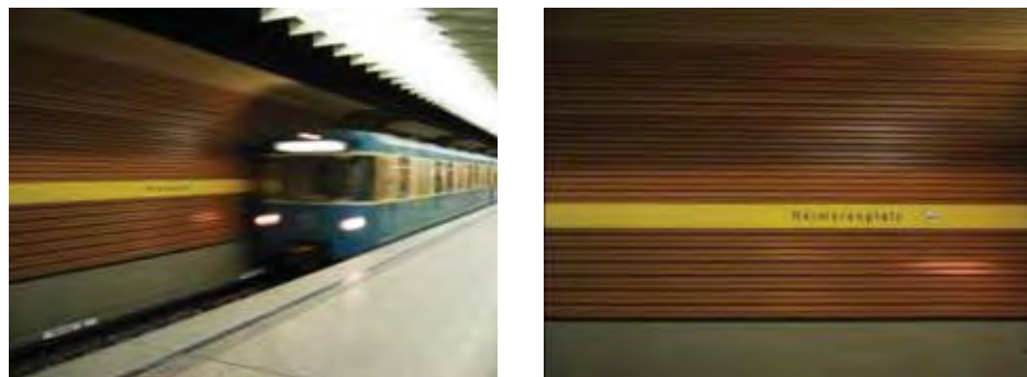
Figure 4-9: Acoustical Panels (Slit And Stat System) Heimeranplatz Station, Munich.‡
