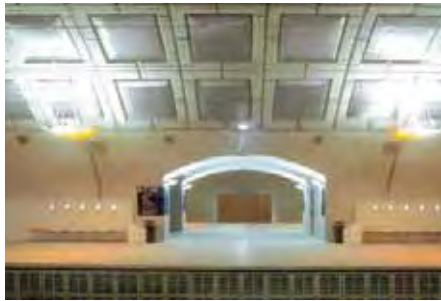
Figure 4-33: Left- Magenta Station With Acoustical Ceiling Treatment And Noise-Absorbent Baffles Between Tracks Magenta Station.
