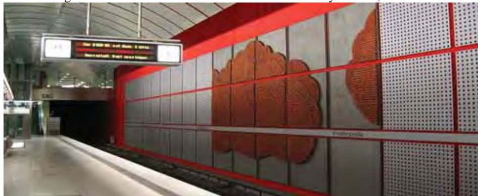
Figure 4-8: Perforated Panels Kreillerstraße Subway Station, Munich.†
