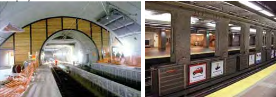
Figure 4-14: Left - Barriers Between Tracks. Downtown Crossing Station, Boston.*
