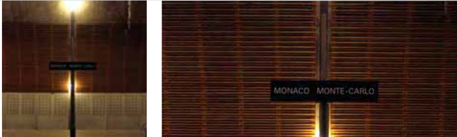
Figure 4-16: Acoustical Panels (Slit And Stat System) Monaco Station.*
