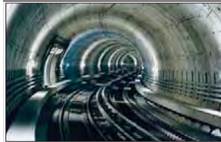
Figure 1-5: Completed Bored tunnel between Attaba and Naguib Stations, Downtown Greater Cairo.*
