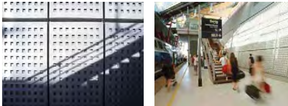
Figure 4-22::Left-Detail, The Angled Platform Walls, Openwork Cement-Glass Composite Panels Are Used In Conjunction With Rockwool(Valence TGV) †
