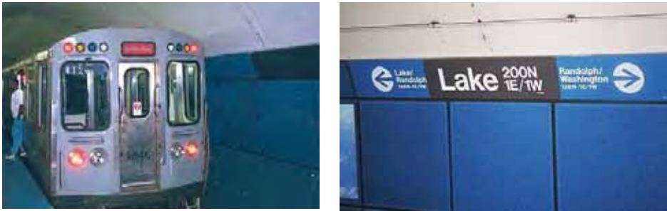
Figure 4-10: Acoustical Panels Fixed Directly On Tunnel Walls. Lake Station, Chicago.*
