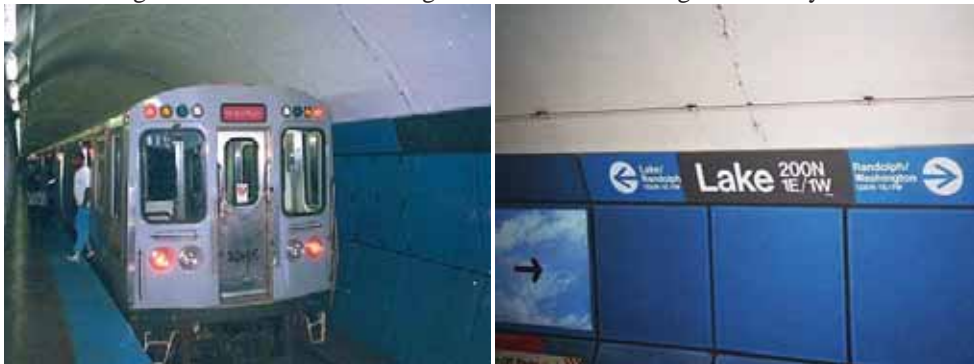
Figure 4-58: Left –Acoustical Treatments In Lake Station. Blue Line, Chicago, USA.
