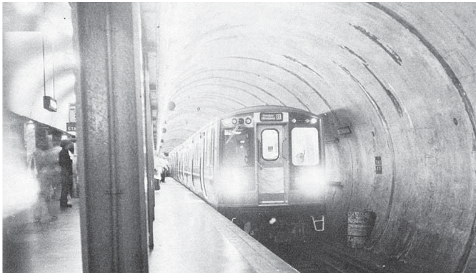
Figure 4-57: Untreated Underground Station In Chicago Transit System
