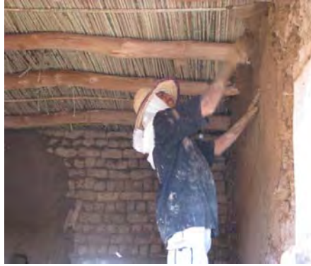
Figure 5.30 Plastering layer is thrown on the walls.
