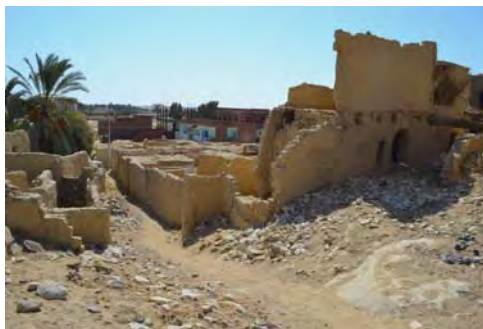
Figure 1.5 Deterioration of vernacular houses and replacement with concrete skeleton ones in the Farafrah oasis.
