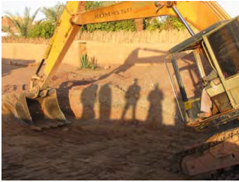
Figure 5.15 The site while digging.
