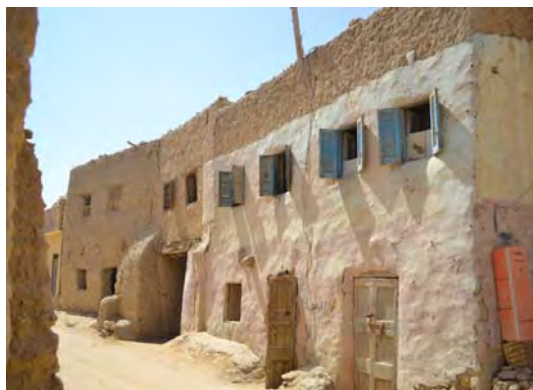
Figure 2.4 A mud brick house in the Farafra oasis. There are similarities but also distinctions between the houses in Baharia, Farafra and Siwa.
