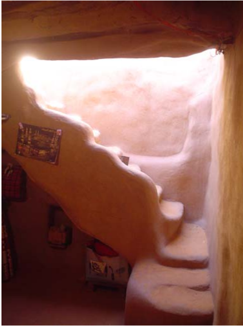
Figure 4.13 Staircase shaft function as wind catchers.
