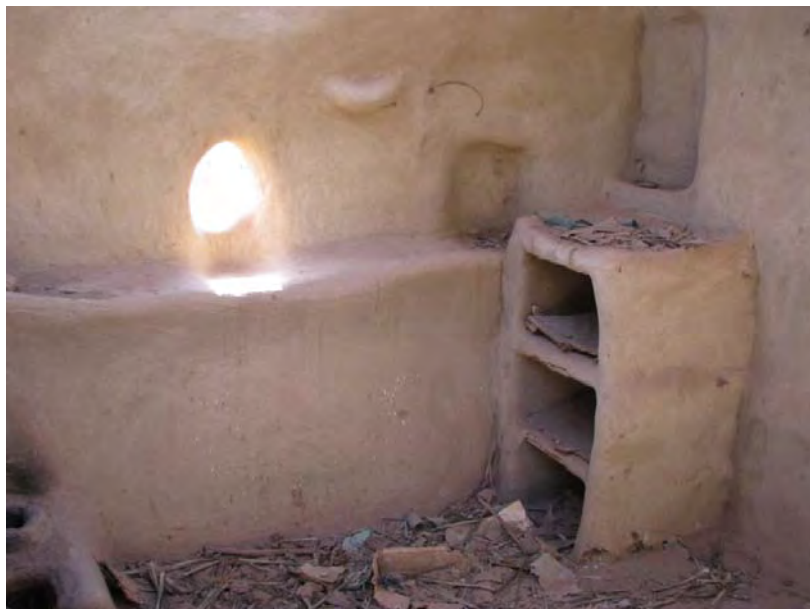
Figure 4.33 Examples of furniture, curved smooth walls, and of an opening made of clay in a deserted house.
