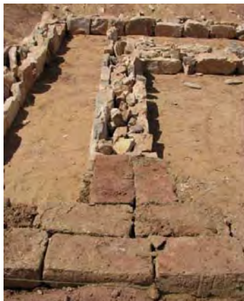
Figure 5.21 The stone and brick footing.
