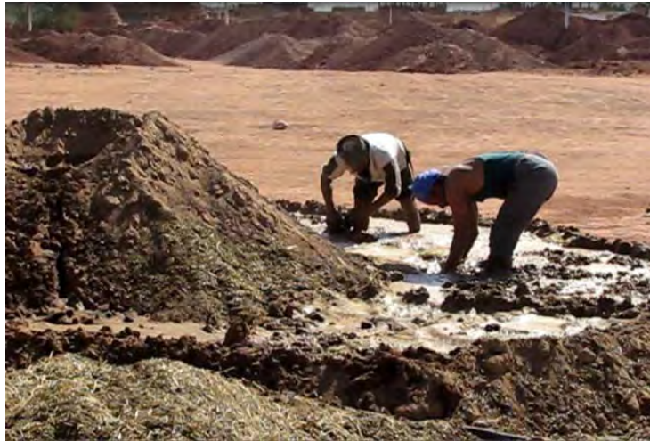
Figure 5.10 Preparing mud, straw, manure, and water for brick casting.
