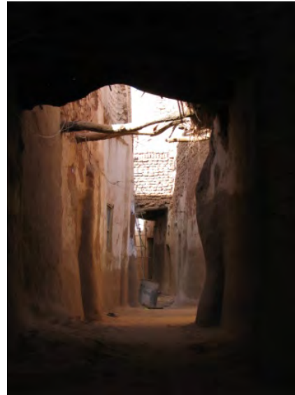
Figure 2.6 Tunnelled shaded streets with light shafts.
