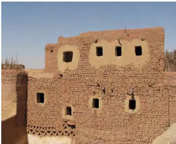
Figure 4.15 Different windows / openings in Balat houses.
