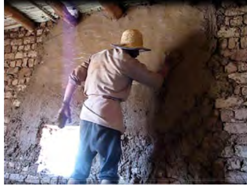
Figure 5.31 Plastering layer is smoothen by wet hand.
