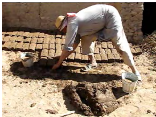
Figure 2.19 Locals in the Dakhla oasis casting mud bricks for restoration work.
