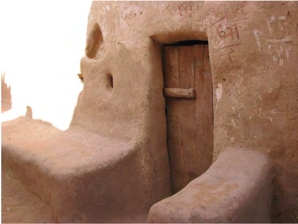
Figure 4.24 Built-in mud brick benches with small niches for candle lamps carved smoothly in walls.
