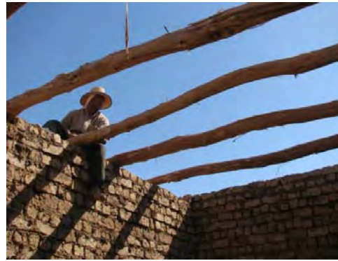
Figure 5.26 Placing the wood logs on the walls.
