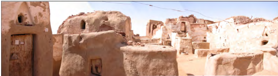
Figure 4.25 Roof floor with several rooms built as mud sculptures.
