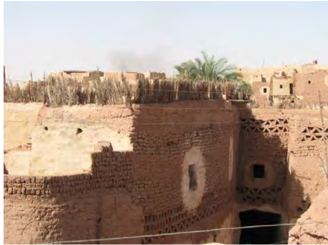
Figure 4.51 Fences around the roof floor made from long palm tree branches.
