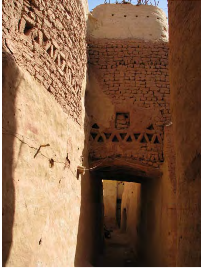
Figure 2.30 A room bridging a street (Sabat). An example of the possibility of making a house extension covering a public alley based on the local civic and Sharia rules ('Urf) within this settlement. The town of Balat in the Dakhla oasis.
