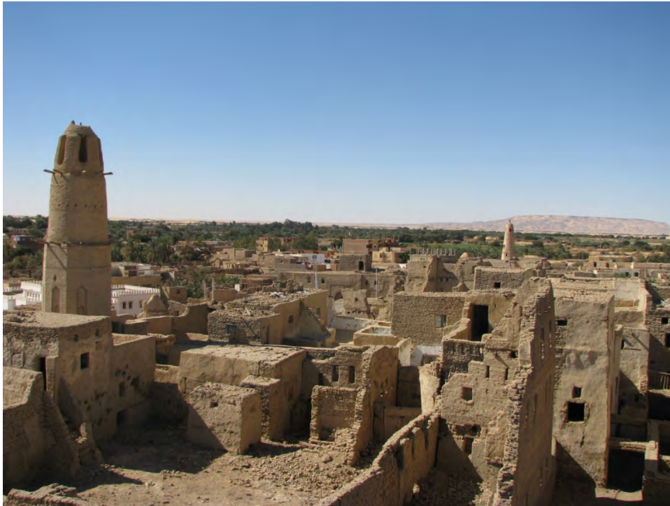
Figure 2.31 Example of a compact structure of a desert vernacular settlement with farm lands and cemeteries lie on the outskirts of Al Qasr town in the Dakhla oasis.
