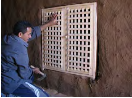
Figure 5.36 Local carpenter while hanging the cabinet door inside the room.
