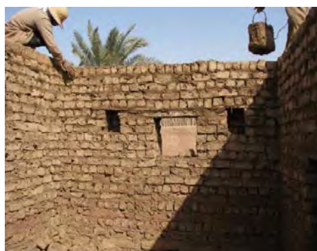
Figure 5.24 Windows and niches during wall construction.
