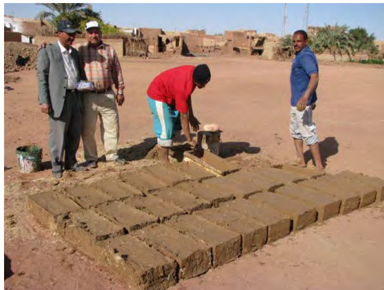
Figure 5.13 Mud brick casting using the second alternative of the mould. Youth were responsible for mud casting in shifts following seniors' instructions.
