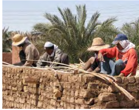
Figure 5.28 Placing palm leaves on top of reeds.
