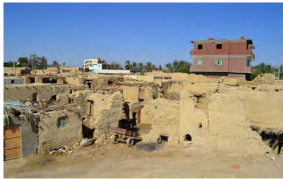
Figure 1.1 Deterioration of vernacular architecture and replacement of Karshif (salt rocks and clay) vernacular houses with concrete skeleton and fired brick ones in the Siwa oasis.
