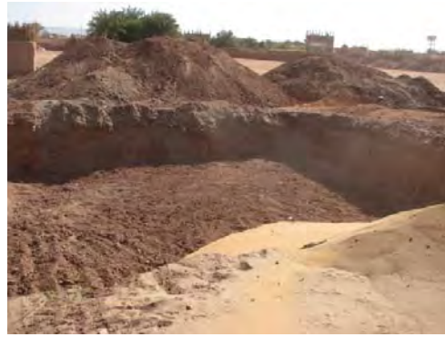
Figure 5.16 The site after digging.
