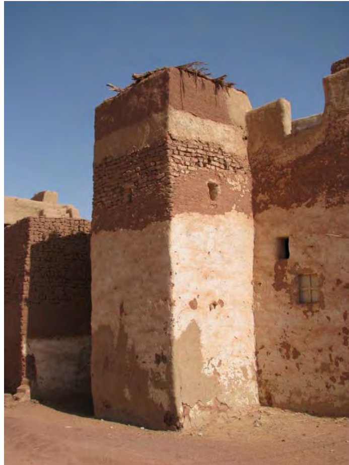
Figure 4.53 Dry toilet (compost) with roof covering from palm ribs and leaves for shade. The toilet has an opening in the bottom of this tower to collect the wastes when they are completely dry twice a year. The wastes are used as soil fertilizers or fuel for ovens.
