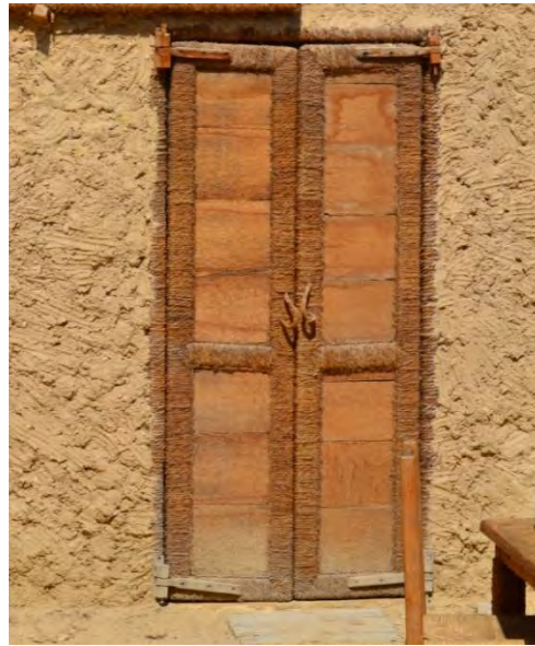
Figure 2.35 Doors in the Siwa oasis made from building construction palm wood leftovers and the door frame and door lock are made from ropes made from palm tree raffia fibers.
