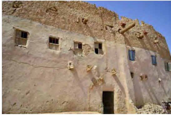
Figure 2.2 A mud brick house in the Siwa oasis.
