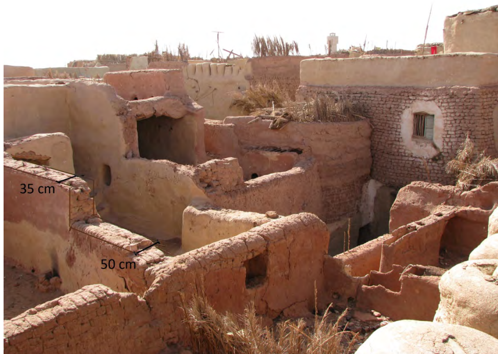
Figure 4.16 Cluster of houses in Balat showing the wall thickness of a second floor and a roof floor.
