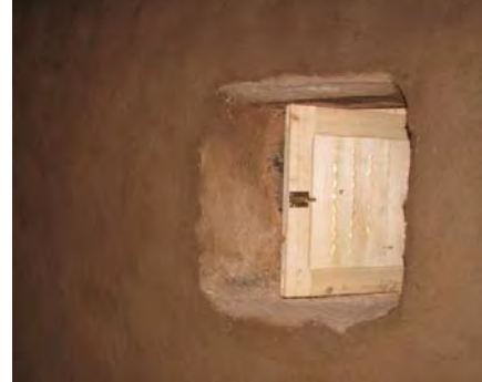
Figure 5.37 The window designed by Balat inhabitants and made by a local carpenter.
