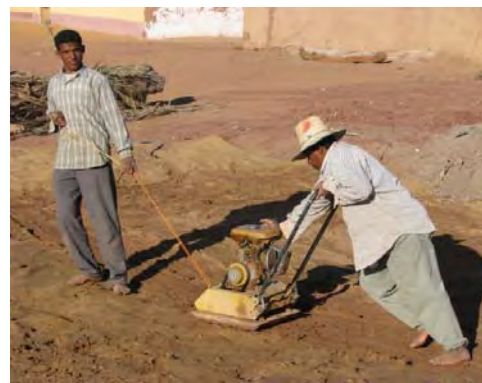
Figure 5.18 The site during soil replacement and compaction.
