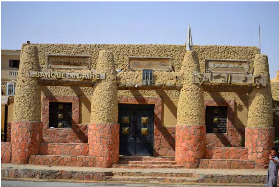
Figure 2.16 Local bank branch designed and constructed by The Siwa Sustainable Development Initiative with earth vernacular building technology in the Siwa oasis using Karshif. According to the designer, the building passed safety and security bank tests in 2008.
