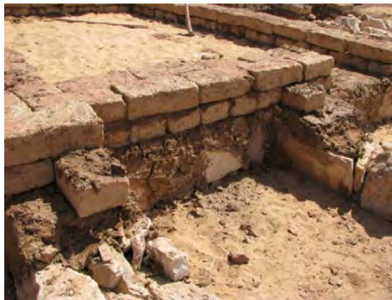
Figure 5.22 Lime is mixed into the footing mortar.
