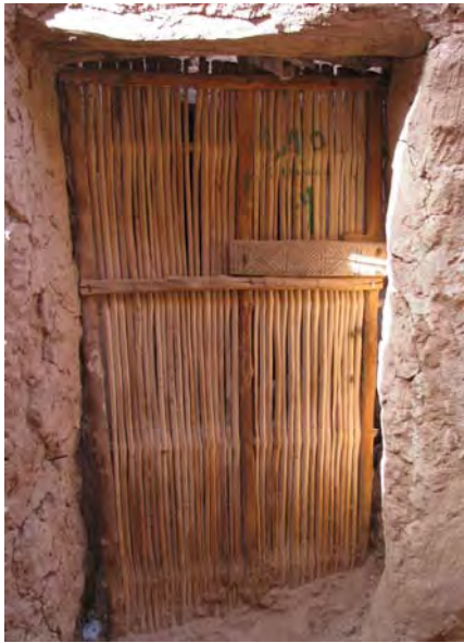
Figure 2.34 Doors in the Dakhla oasis made from palm tree ribs or reeds and the wooden key and lock are made from building construction wood leftovers.
