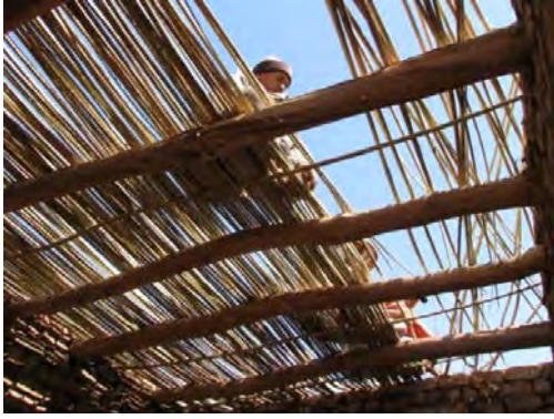
Figure 5.27 Palm reeds placed in a perpendicular manner over casuarina logs.
