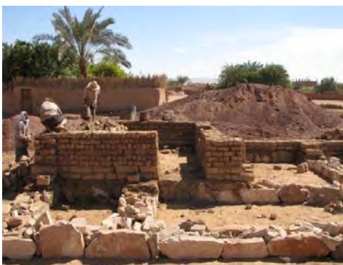
Figure 5.23 Wall construction phase.
