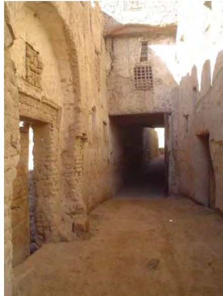
Figure 2.28 Shaded building facades in the Dakhla oasis.
