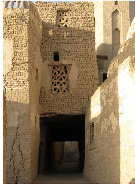
Figure 5.4 Shaded alley and a room bridging a street (Sabat) in Al Qasr in the Dakhla oasis.
