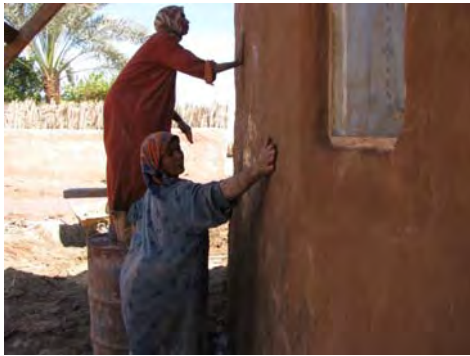
Figure 5.32 Exterior wall rendering with the help of Balat ladies using traditional manual techniques.
