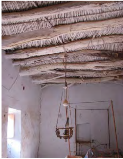
Figure 4.89 Roof structure made from acacia wood logs and palm ribs.
