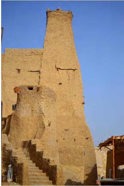
Figure 5.1 A mosque minaret in the Siwa oasis.
