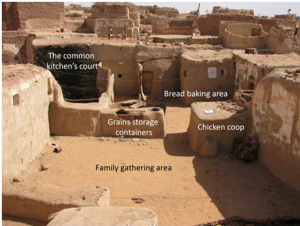
Figure 2.33 A floor constructed on a roof in order to extend a house, with four families sharing facilities such as a common kitchen, chicken coop and wheat storage, Dakhla oasis.
