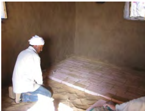
Figure 5.34 Floor making using sand tiles.
