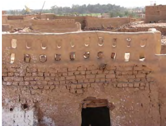
Figure 4.50 Example of exterior fences (parapets) in the roof floor made from mud brick .
