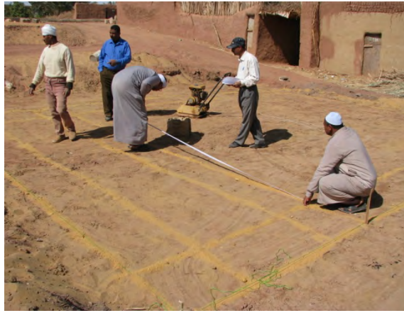
Figure 5.19 Drawing the house plan on the ground using the vernacular way.
