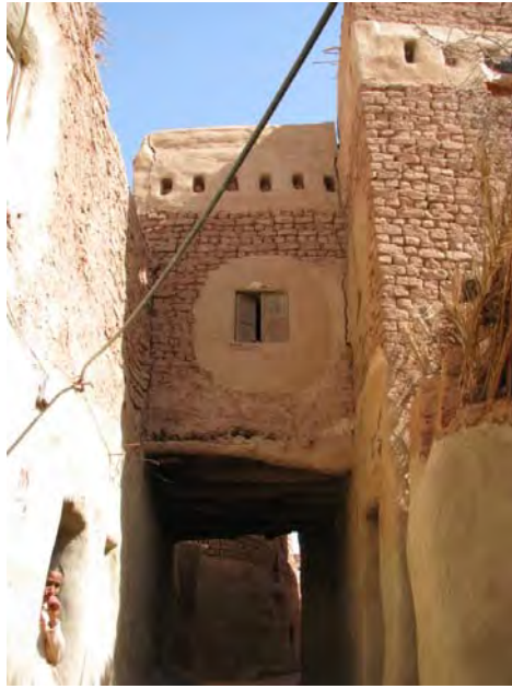
Figure 5.3 Shaded alley and a room bridging a street (Sabat) in Balat in the Dakhla oasis.
