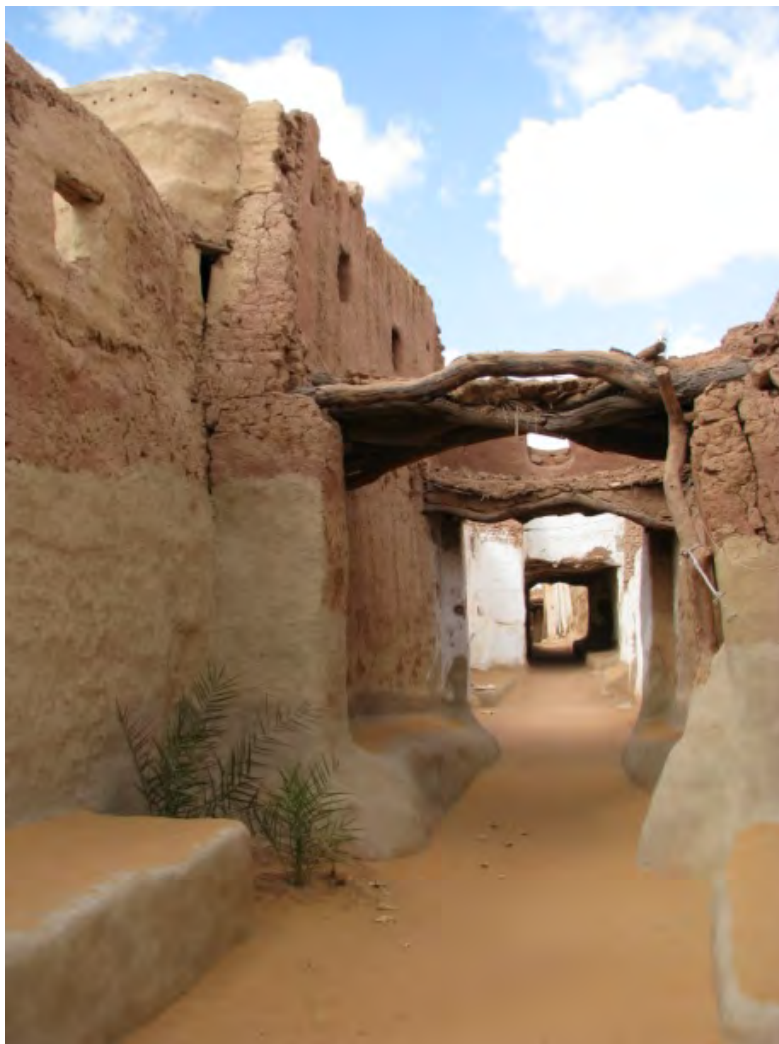
Figure 4.23 Built-in mud brick benches (Mastaba) is a main feature in the streets in Balat. They add an aesthetic touch to the townscape.
