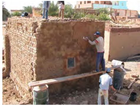
Figure 5.33 Exterior wall rendering using plastering trowels.
