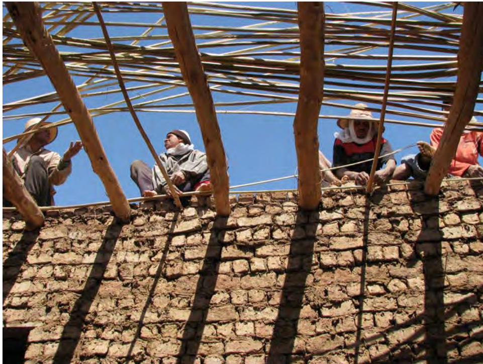
Figure 2.20 Traditional roof structure making process in the Dakhla oasis.
