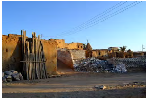
Figure 1.2 Deterioration of vernacular architecture and replacement of vernacular houses with concrete skeleton and white brick ones in the Baharia oasis.
