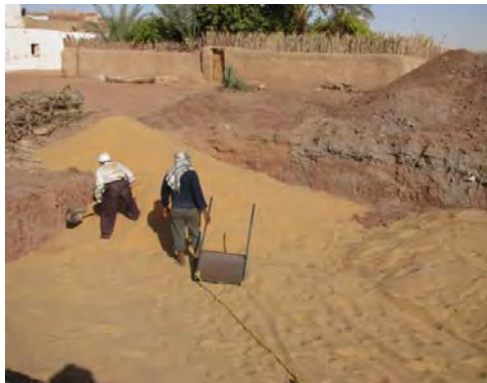
Figure 5.17 The site during soil replacement with fresh sand layers.
