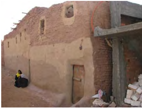
Figure 1.3 Replacement of mud brick vernacular houses with concrete skeleton ones in the Dakhla oasis.
