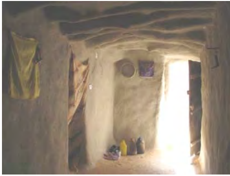
Figure 2.38 A room before monthly regular maintenance in the Dakhla oasis.
