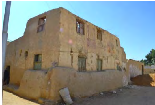
Figure 2.3 A mud brick house in the Baharia oasis.
