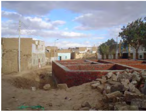
Figure 1.4 Replacement of mud brick vernacular houses with concrete skeleton ones in the Kharga oasis.
