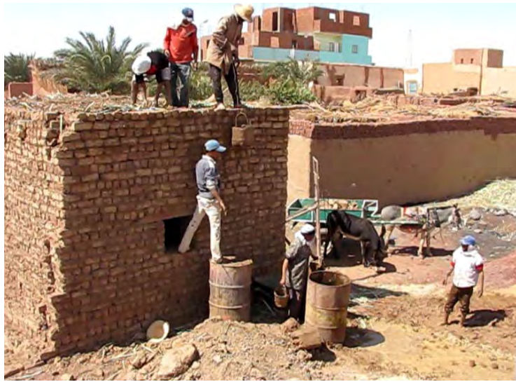
Figure 5.29 Applying the mud brick and the mortar layers.
