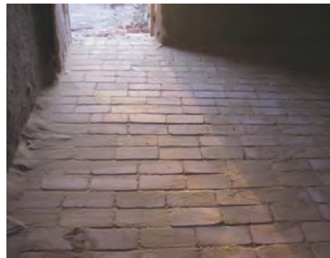
Figure 5.35 Sand floor tiles after finishing.
