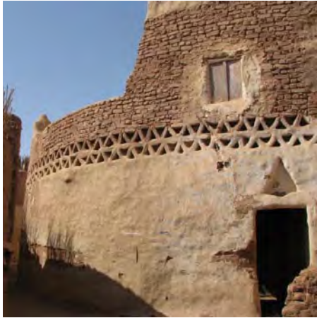
Figure 2.23 Smooth curved building corners in the Dakhla oasis.
