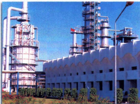
Distillation Columns Building (DCS) (Fractionator)
