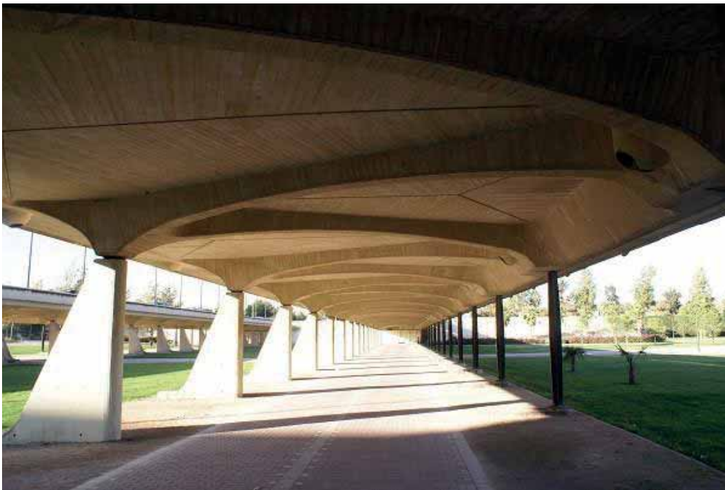
Fig. 1.42: 9th of October Bridge in Valencia.
