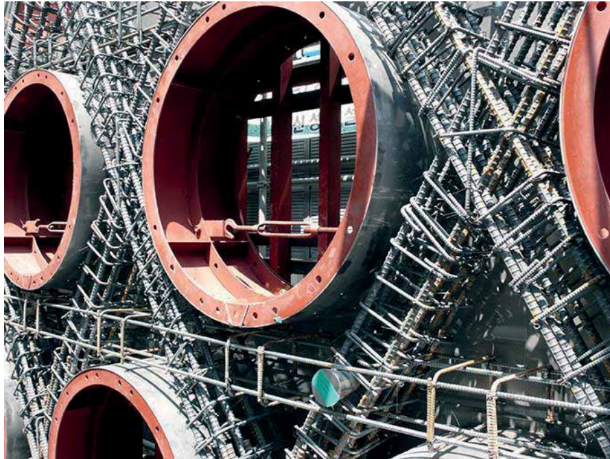
Fig. 4.30: Reinforcement during Construction.
