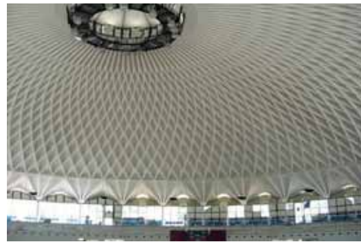
Fig. 1.41: Palazetto dello sport dome ribs.
