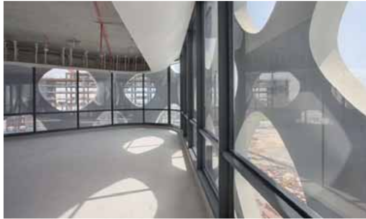
Fig. 4.24: Column Free Interior Space.
