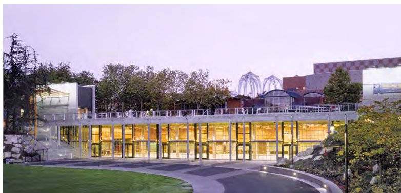
Figure (4-33) The Northern Glazed Façade of Seattle Center-Fisher Pavilion. ( www.millerhull.com/htm/nonresidential/SeattleCenter.htm )
