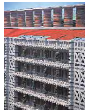
Figure (a-14) Eastgate Center Exterior Shows the Chimneys and Photovoltaics
