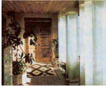
Figure (4-40) Thermal Water Wall in Small Office in New Mexico. (Anderson and Wells, 1981)
