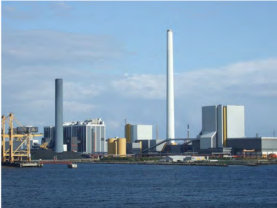
Figure (1-11) The Industrial Ecosystem at Kalundborg. View from Around the Asnaes Power Station ( www.kythuatvatlieu.org/definition/categories.html?view=mediawiki&article=File%3AView_from_Asnaes_power_station_Kalundborg_Denmark.jpg )
