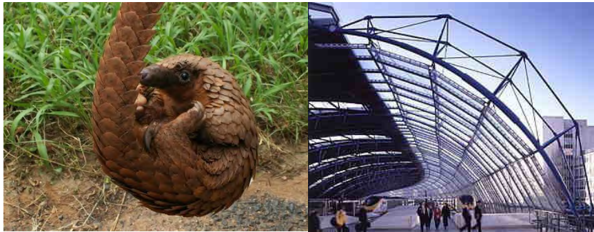
Figure (1-62): Waterloo International Terminal Covering Joints after the Pangolin Flexible Joints.
