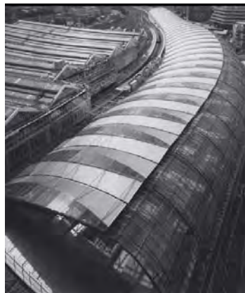
Figure (a-24) Waterloo Terminal Exterior. ( www.owlnet.rice.edu/~arch214/waterloo.pdf )
