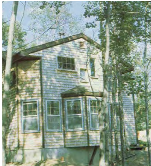
Figure (4-35) Bow Window Maximizes Heat Gain in a Low Energy House Façade. (Anderson and Wells, 1981)
