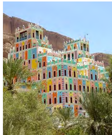
Figure (4-8) Multistorey Arrangements Reduce Exposed Envelope Area.
