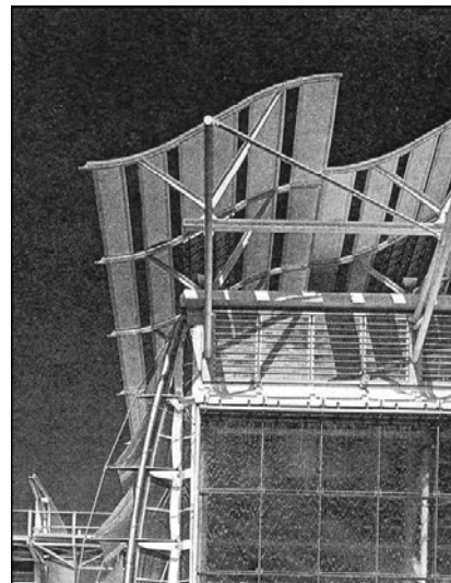
Figure (a-30) Solar “Hats” on the Roof of the British Pavilion at EXPO 1992. (Todorovic, 2005)
