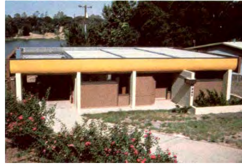
Figure (4-41) A House in Atascadero, California with Water Solar Roof. (Anderson and Wells, 1981)
