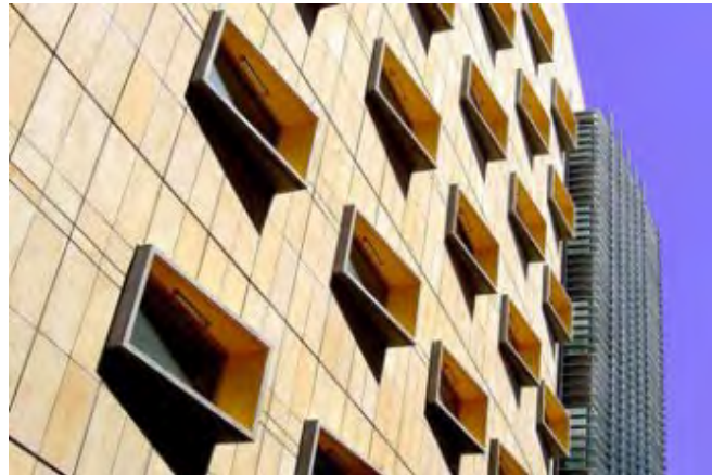
Figure (4-22) Assymetry in Sun Breakers Orientation in USEK Student Housing in Lebanon
