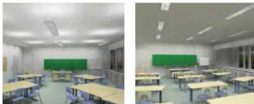
Figure 3- 11: Indirect luminaire is better in smart learning spaces with movable furniture Source: Good Lighting for Schools and Educational Establishments, p. 5
