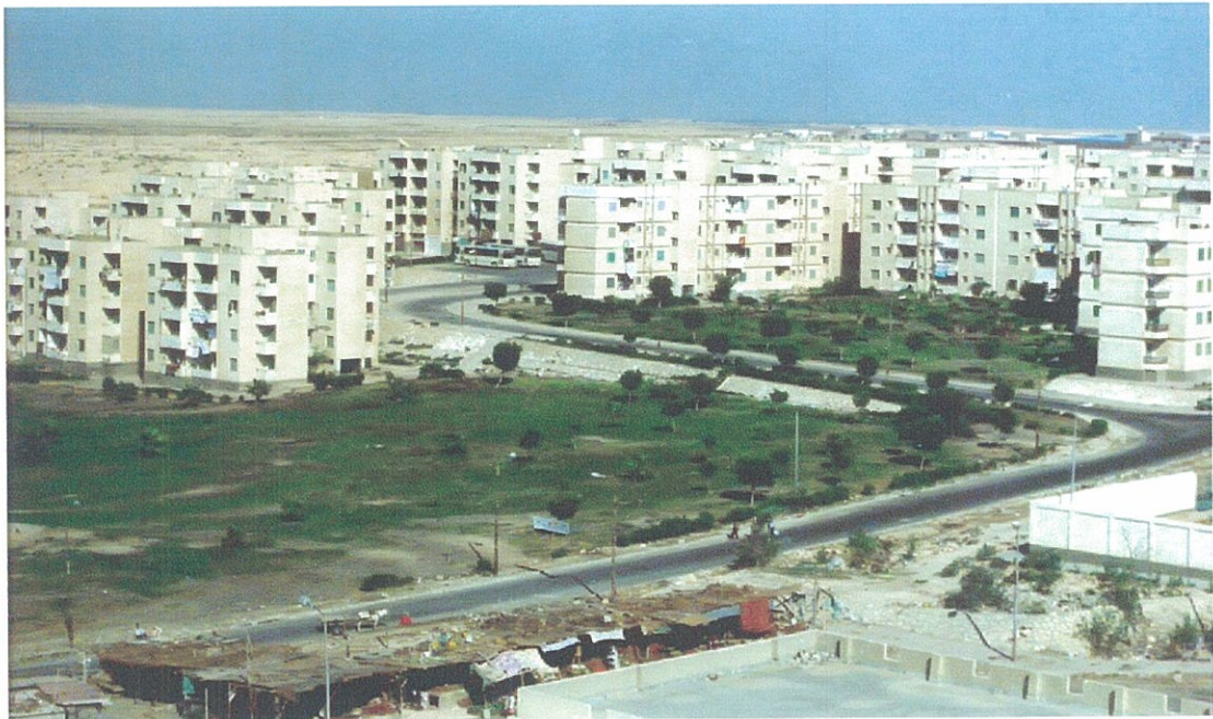
The Residential Zone and the Wednesday Market (at the bottom) [a green belt separates the residential zone from the Market]
