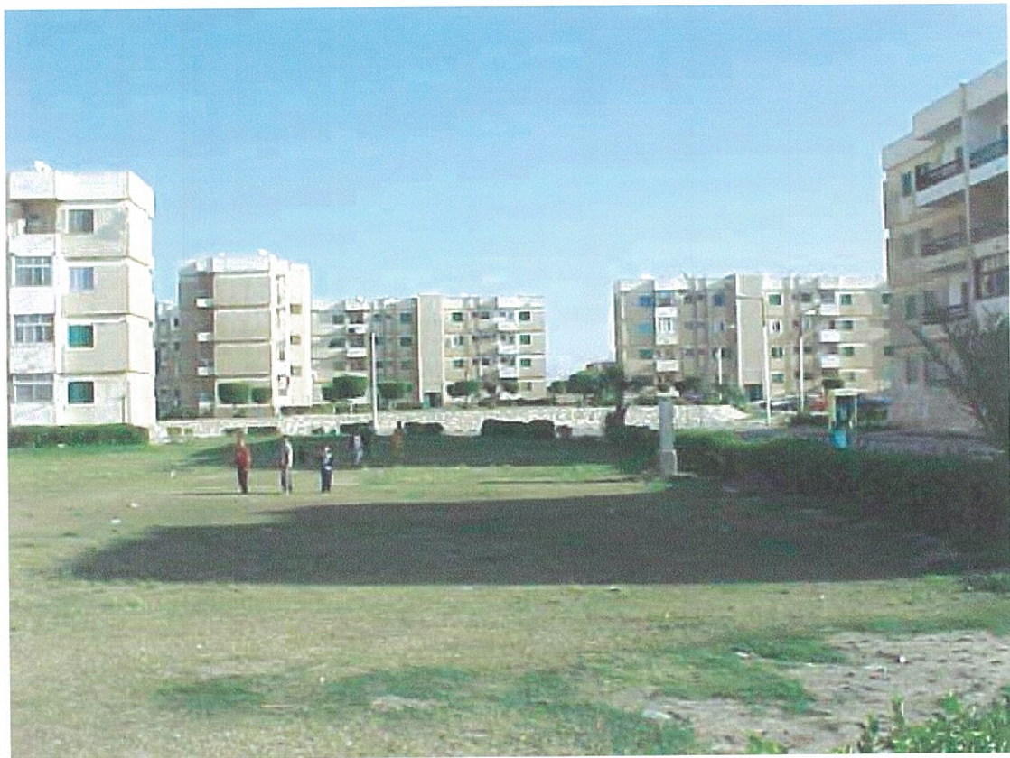
Wide Green Areas between Residential Blocks
