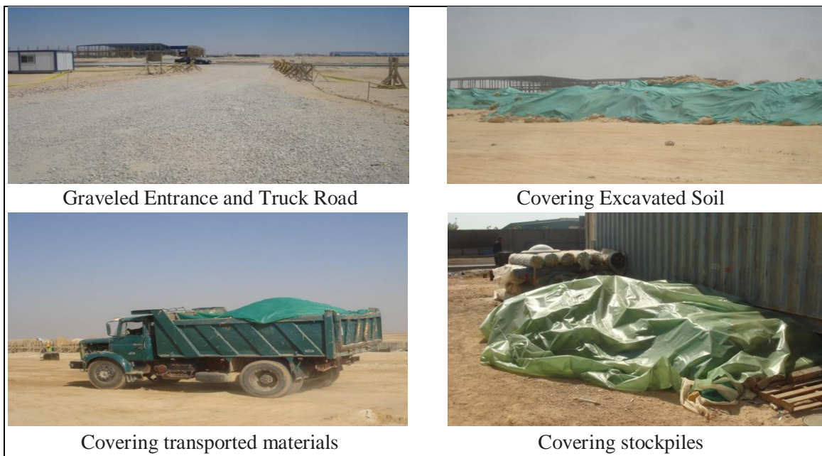
Figure 4-2 : Sample of photos presented in the ESC Plan which is submitted as a part of the documentation for SSp1
