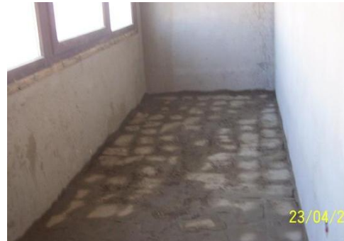
Reusing of hollow blocks waste on site
