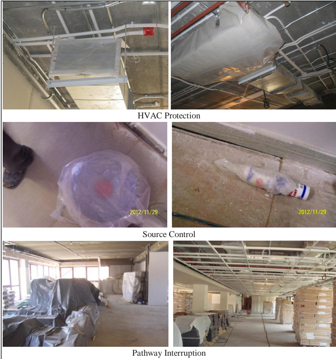
Figure 4-12: Sample of photos presented in the IAQ Plan during construction which is submitted as a part of the documentation for IEQc3.1
