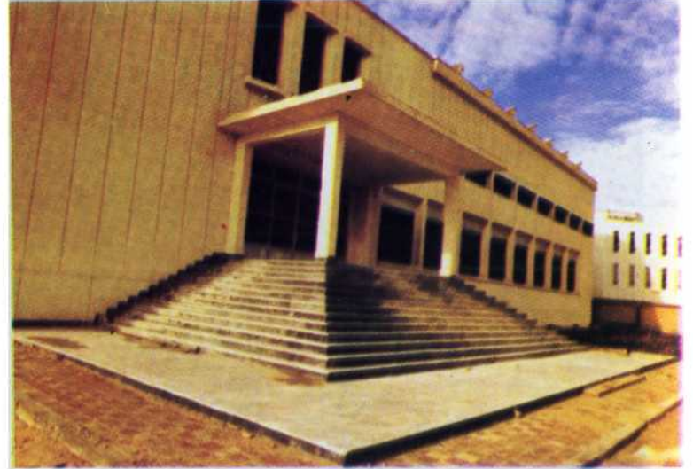
• The eastern elevation of the museum.
