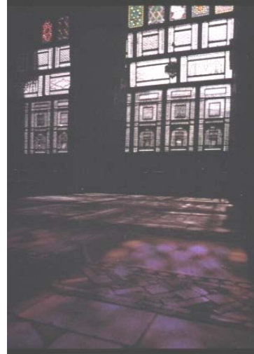
Figure1: A traditional design of “mushrabiyya” adapted to adjust the amount of desired light and air penetrating into the interior space.
