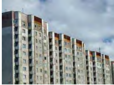
Figure 3.8 Panelised Apartment Block (Csagoly, 1999)
