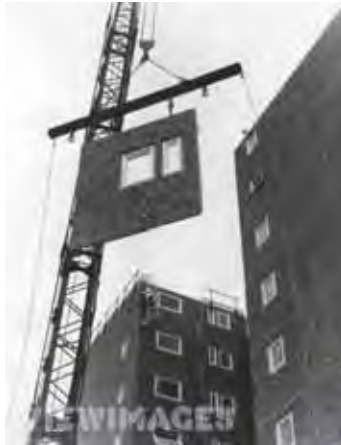
Figure 3.7 Construction of a Precast Concrete Panel House (World Press Photos, 1965)
