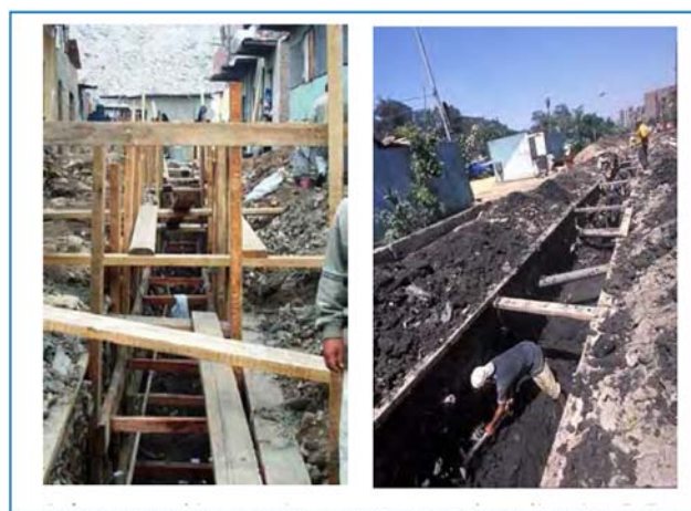
Fig 5; illustrates Infrastructural interventions: sewage network amelioration, BeD. ©GTZ.
