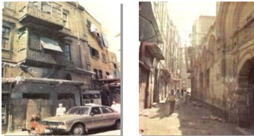
Fig. 6. The deterioration in urban stock of El Moaied Mosque area – Historic Cairo REFERENCES ( 12 ).
