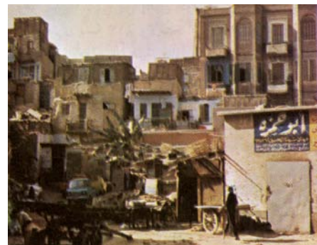
Fig 5, The deteriorated urban areas around the historical building at El Nasr Gate area – Cairo.
