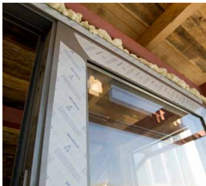
Building retrofit in Kyrgyzstan (EBRD)
