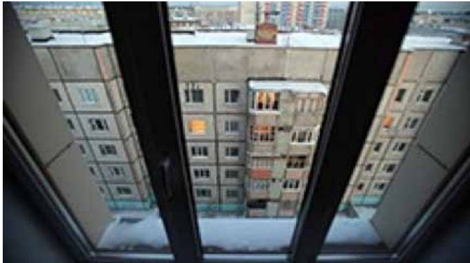
Energy efficiency measures in a building in Western Syberia financed by the EBRD
