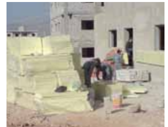
Installation of thermal insulation at MED-ENEC I pilot project in Syria
