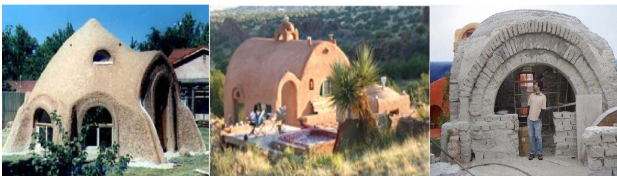
Fig. 6: Paper-Crete - is innovative sustainable building material made of shredded recycled newspaper, water, cement and sand, which harden to form a material that is virtually non-flammable, has high compressive strength and is an excellent insulator. The material can be dyed in the same way as cement and can be painted.
