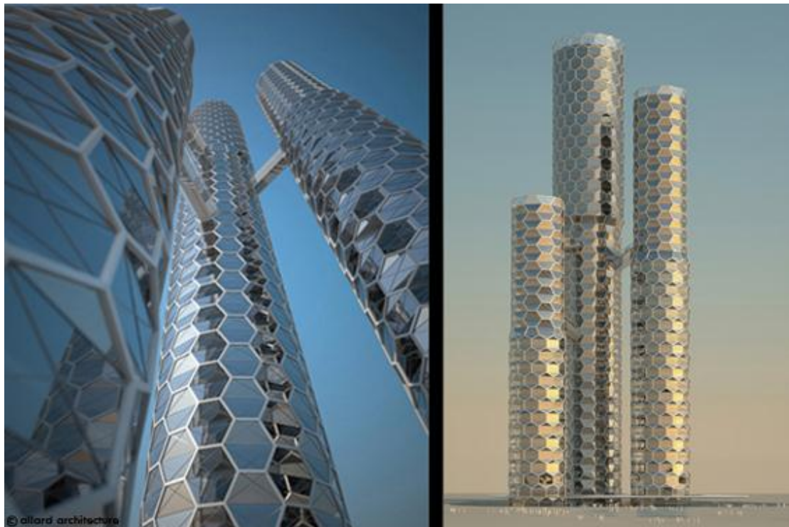
(Fig. 15) The Nano Towers (Proposal), The new headquarters of the DuBiotech Research Park in Dubai, Allard Architecture, (imitating the form of carbon nanotubes)
