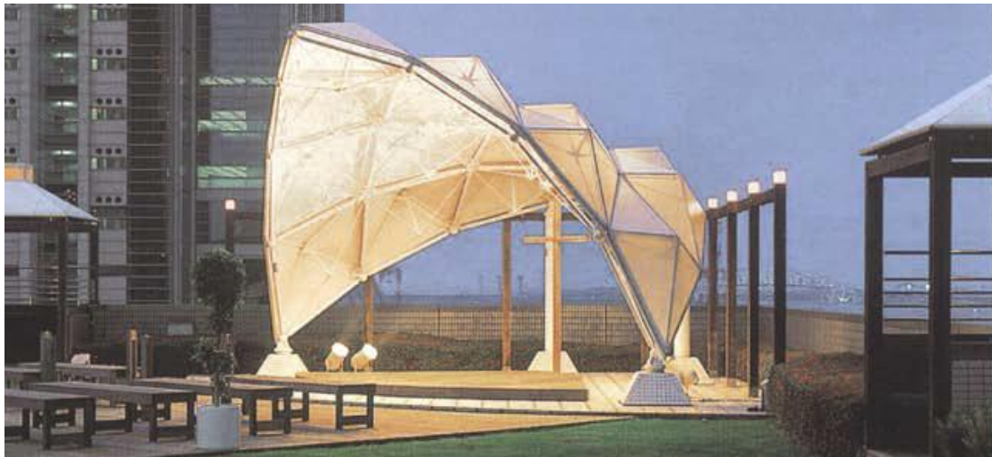
(Fig. 10) Hyatt Regency Osaka Sky Clear Coat fabric/ \text{TiO}_2 photocatalytic self-cleaning membrane [1]
