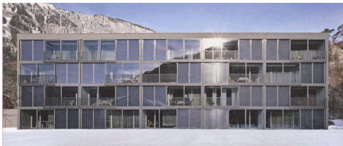
(Fig. 7) "Sur Falveng" house for elderly people, façade, Switzerland
