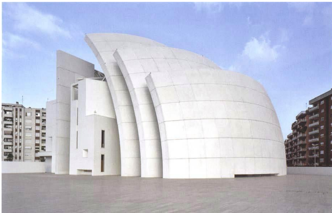
(Fig. 4) Jubilee Church, Rome, Italy, Richard Meier, 2003, (TX Millenium, TX Active, photocatalytic cement) [4]
