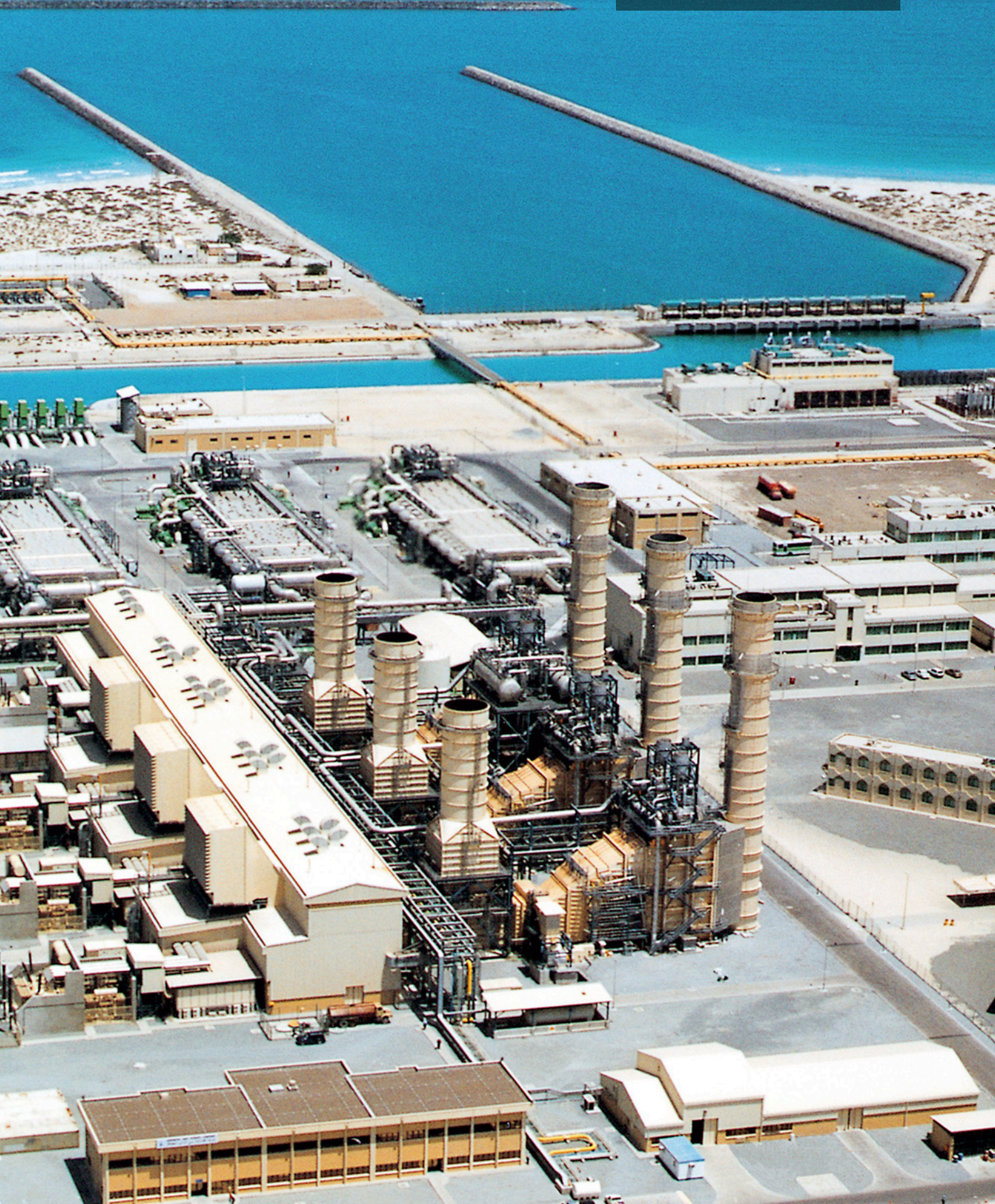
Al Taweelah A2 gas and steam power station and a connected desalination plant in the United Arab Emirates
