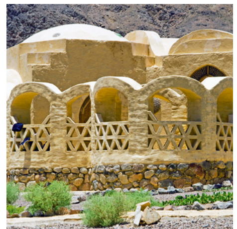
Energy efficient building techniques blended with traditional culture and style at Basata, Egypt
