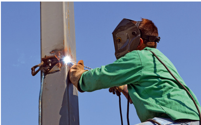
Skilled and semi-skilled construction and manufacturing jobs such as welding will be created through investments in buildings energy efficiency
