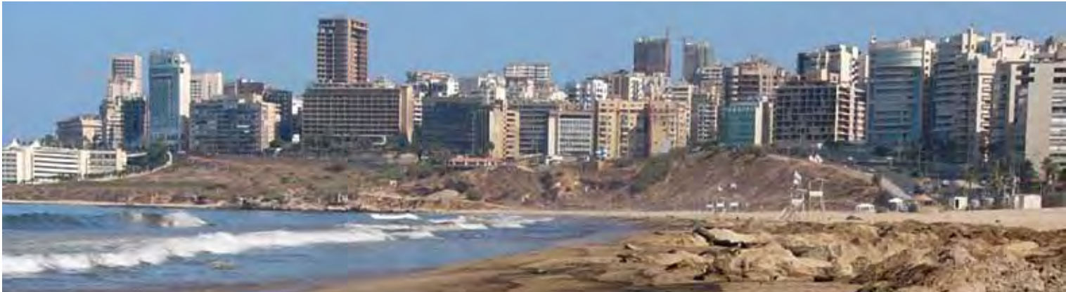
Lebanon: Beirut Skyline documents the mainstream of energy consuming constructions in the MENA region
