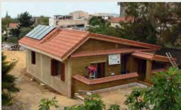
Algeria: MED-ENEC pilot project – EE country house
