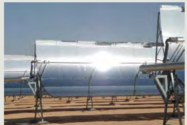
Morocco: Ouarzazate solar power station
