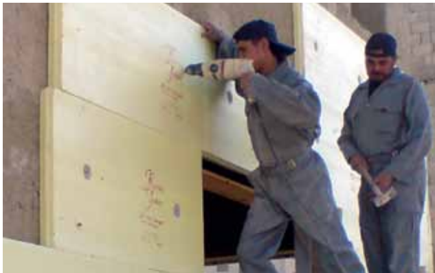
Syria: Installation of insulating wall panels
