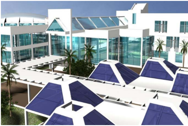
PV units as a part of external shade, new Labs building in 6th Oct. city (1 st prize competition, 2008)
