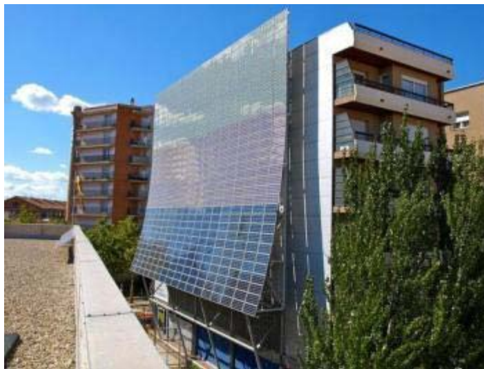
Figure 10: Photovoltaic wall at MNACTEC Terrassa in Spain (Chixoy, Wikipedia, 2013)
