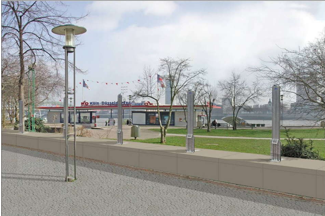
Figure 13 before closing the retaining walls
